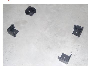
Step 4: place cabinet onto the corner sections and bolt cabinet onto them.
